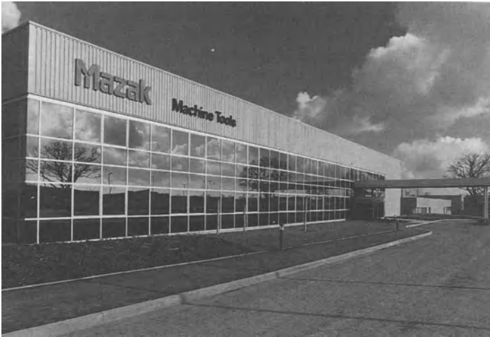
Fig. 2.12. One of the most modern factories in Europe, in Worcester, England. A fully integrated CIM facility, producing 100 machines/month by 240 staff on 14.5 acres. [Courtesy of Yamazaki Mazak Ltd.]
